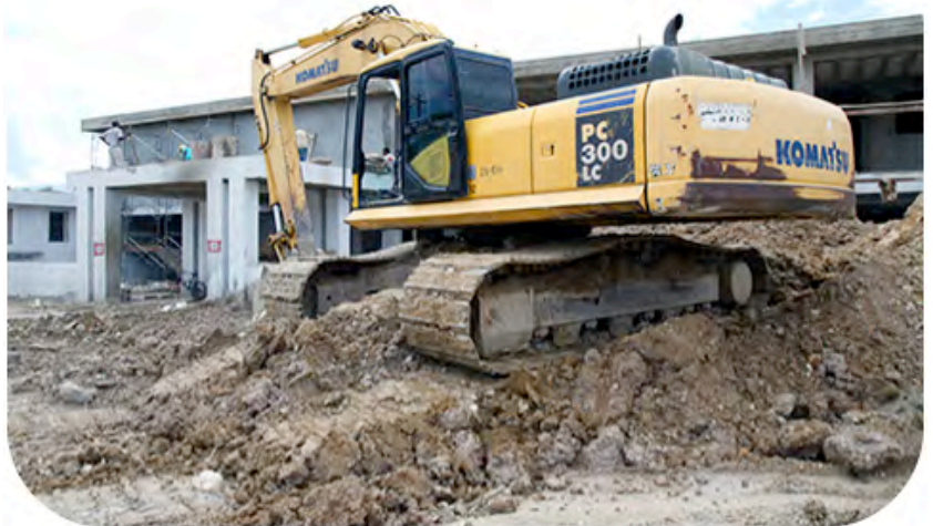
Construction continues on the new Partners In Health hospital in Mirebalais
